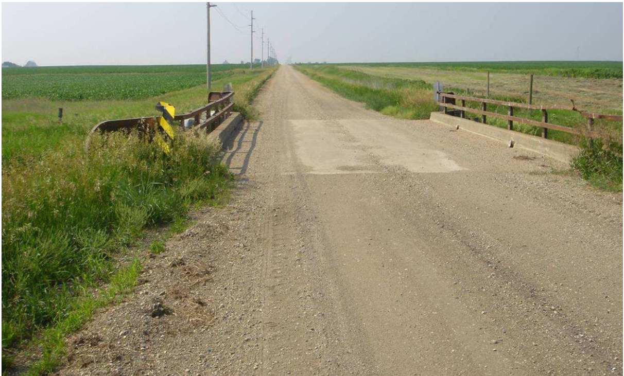
Figure 3.1. BCB Alignment View Looking South.
