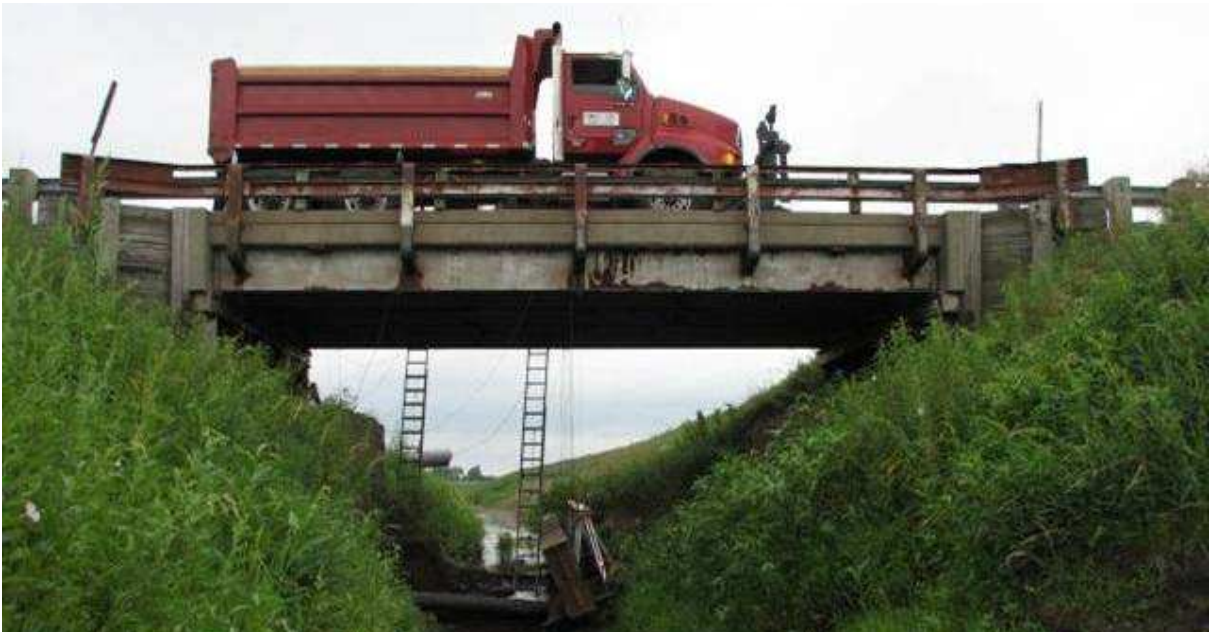
Figure 8.4. HCB Test Truck Crossing Bridge After Pier Removal.
