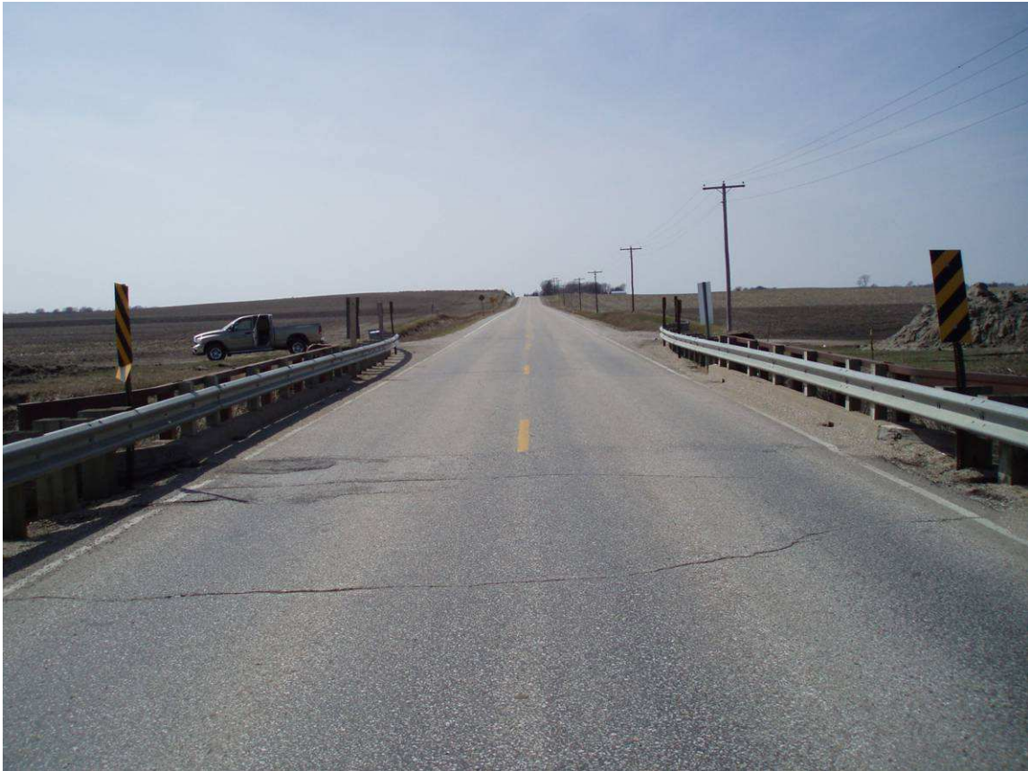
Figure 8.1. HCB Alignment View Looking West.
