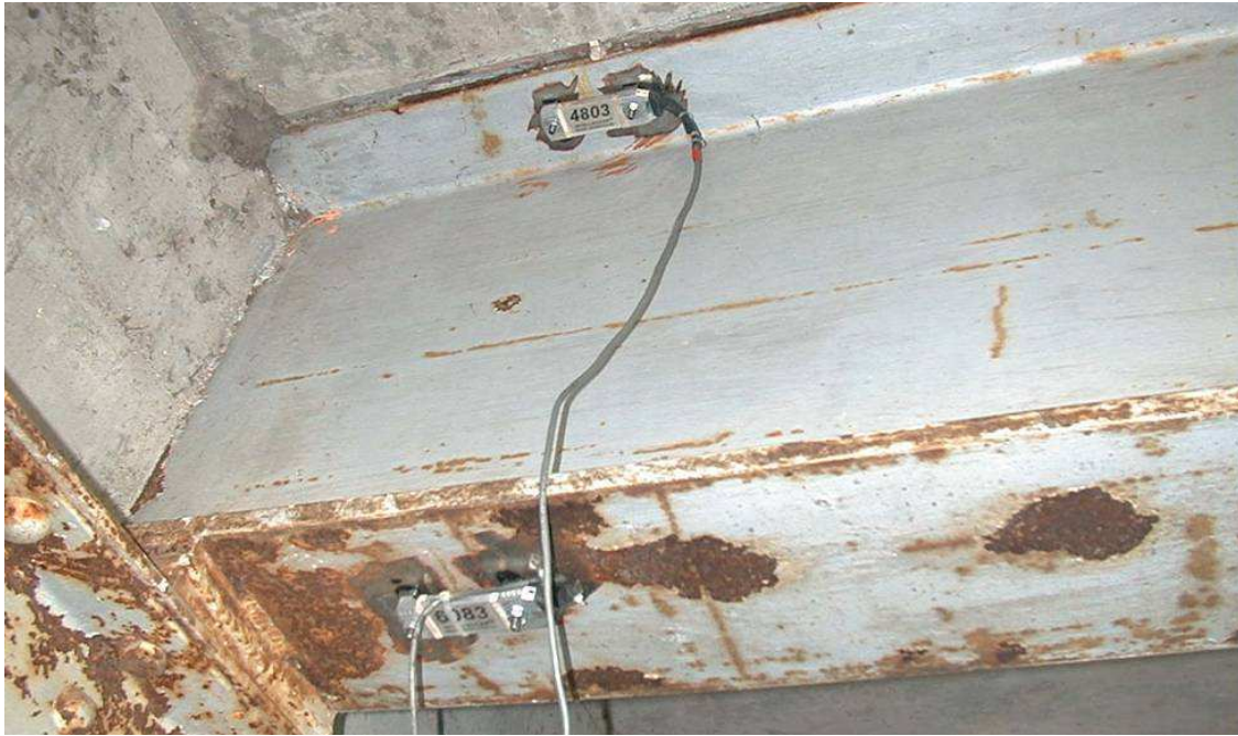
Figure 3.12. Instrumentation Near Abutment of BCB
