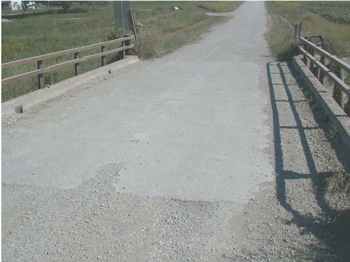
Figure 5.1. KCB1 Alignment View Looking North.
