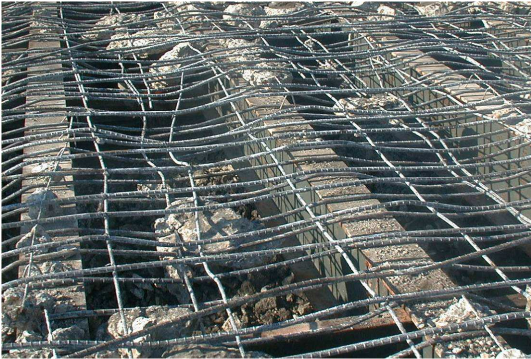
Figure 4.17. Exposed Top Flanges After MCB Deck Demolition.
