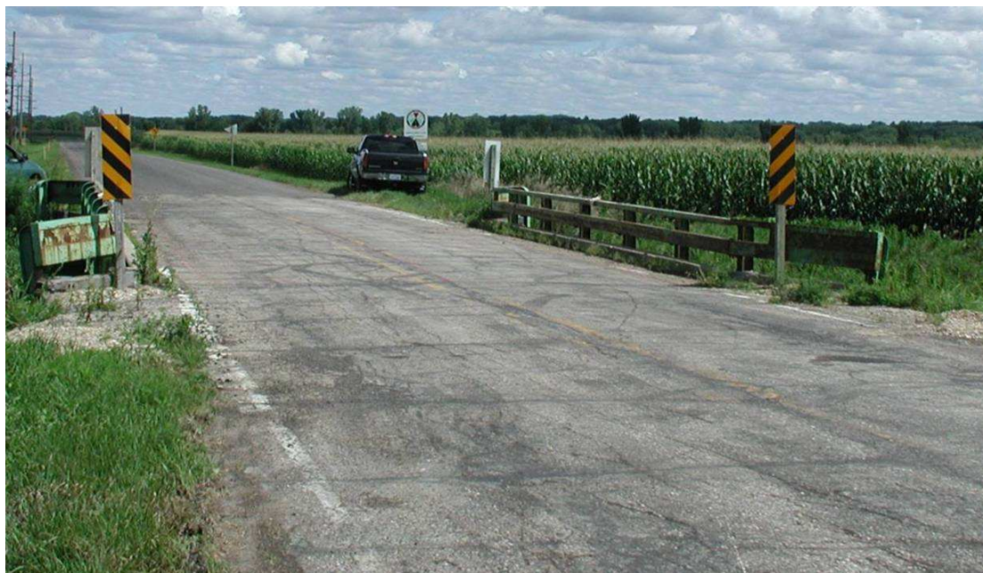
Figure 4.1. MCB Alignment View Looking North.
